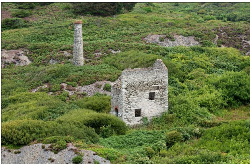
Blue Hills pumping engine house, St Agnes – Photo: Adam Sharpe
